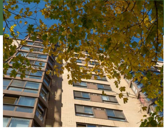
Charles Hastings Housing Co-operative, Toronto, Ont.
