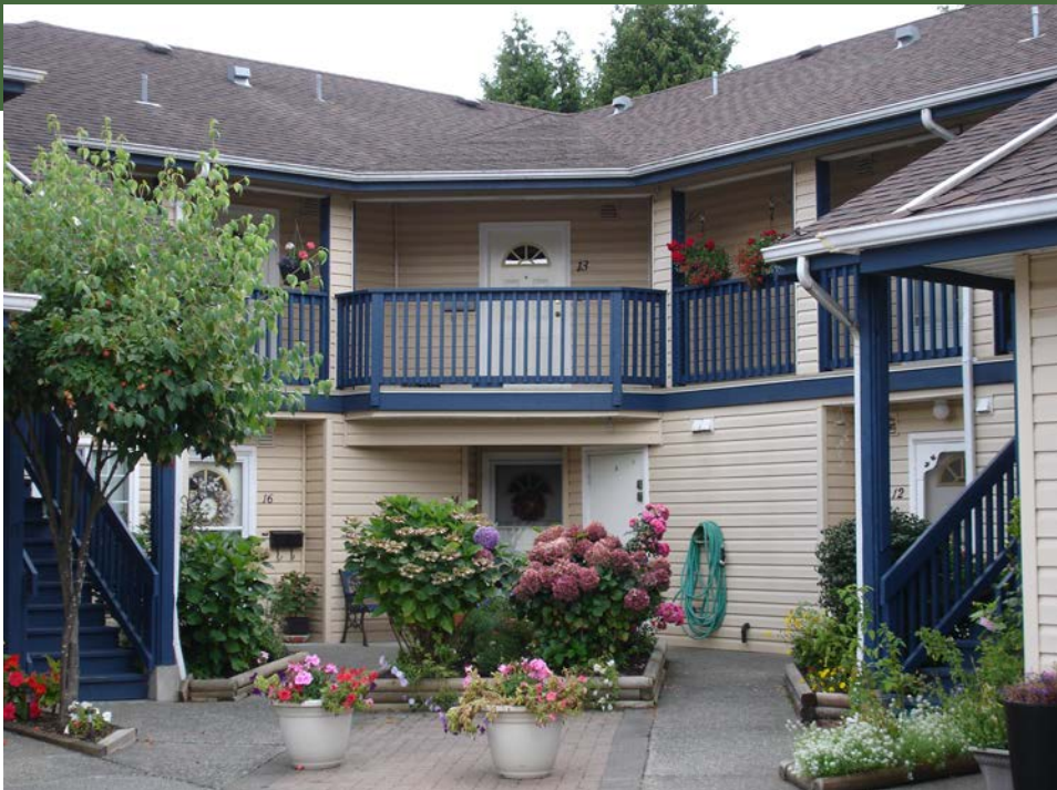
Blueberry Vale Housing Co-operative, Richmond, C.-B.
